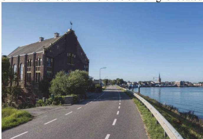
Fig. 2: A church that was build in the dike
